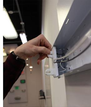
6. Unfasten screws holding down ballast. Remove ballast and sockets at once. Discard according to manufacturer's recommendation.
