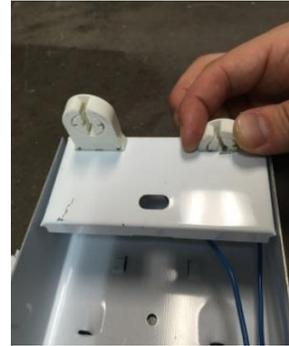
6. Unfasten screws holding down ballast. Remove ballast and sockets at once. Discard according to manufacturer's recommendation.
