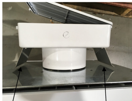
Spring clips hold fixture in place
